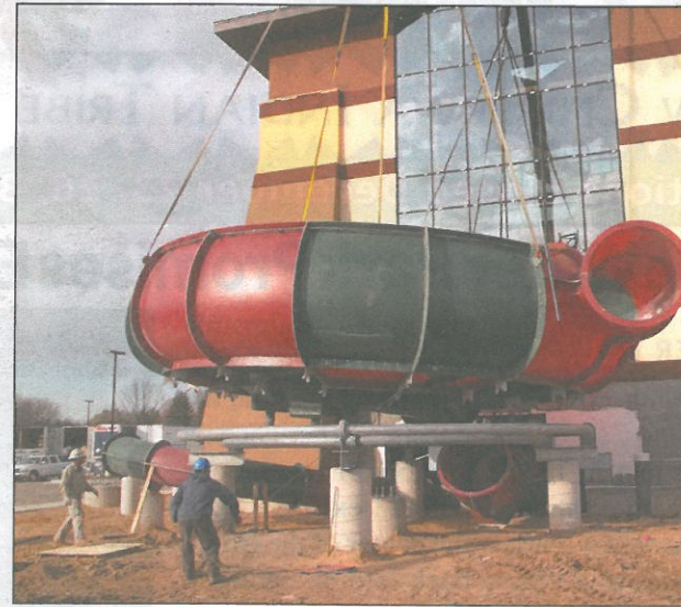
Water bowl being set on it's foundation.
