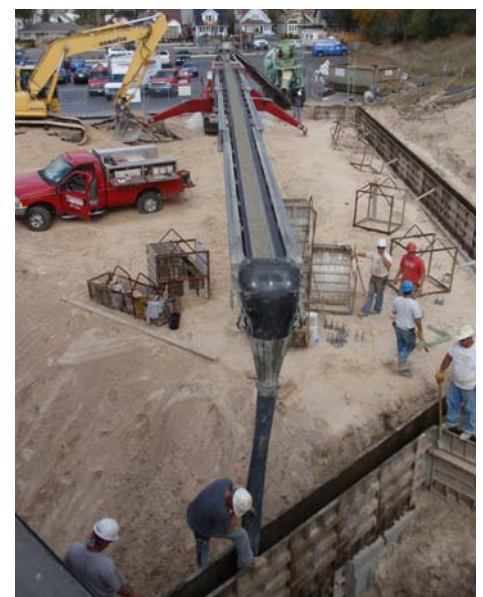
Conveyor belts are used to pour concrete for interior foundation walls.
